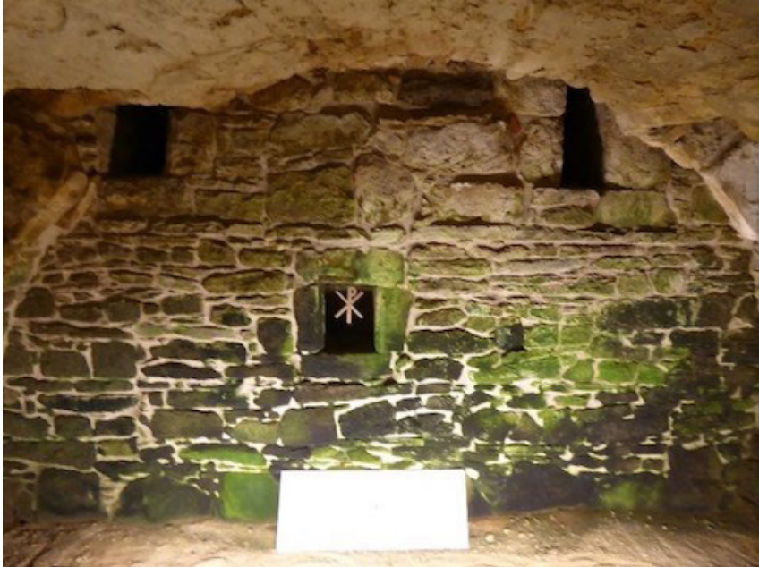
Masonry in the crypt at Portmahomack
